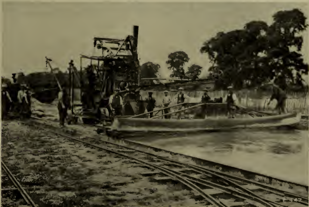
THE CAMBRIDGE ROAD: UNDER CONSTRUCTION.
